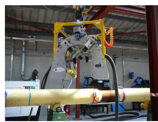
Surface cleaning Grit blasting
