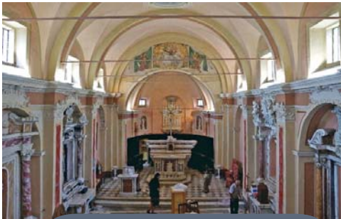
Site photography and measurements
